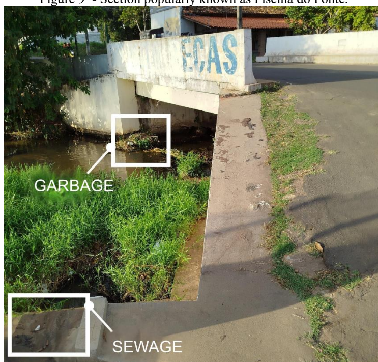
Figure 9 - Section popularly known as Piscina do Ponte.
