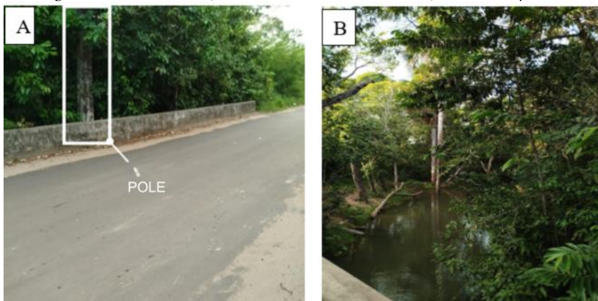
Figure 3 - A: Bridge over the Inhamum stream, in a section known as Cantinho do Céu; B: Preserved riparian forest vegetation.
